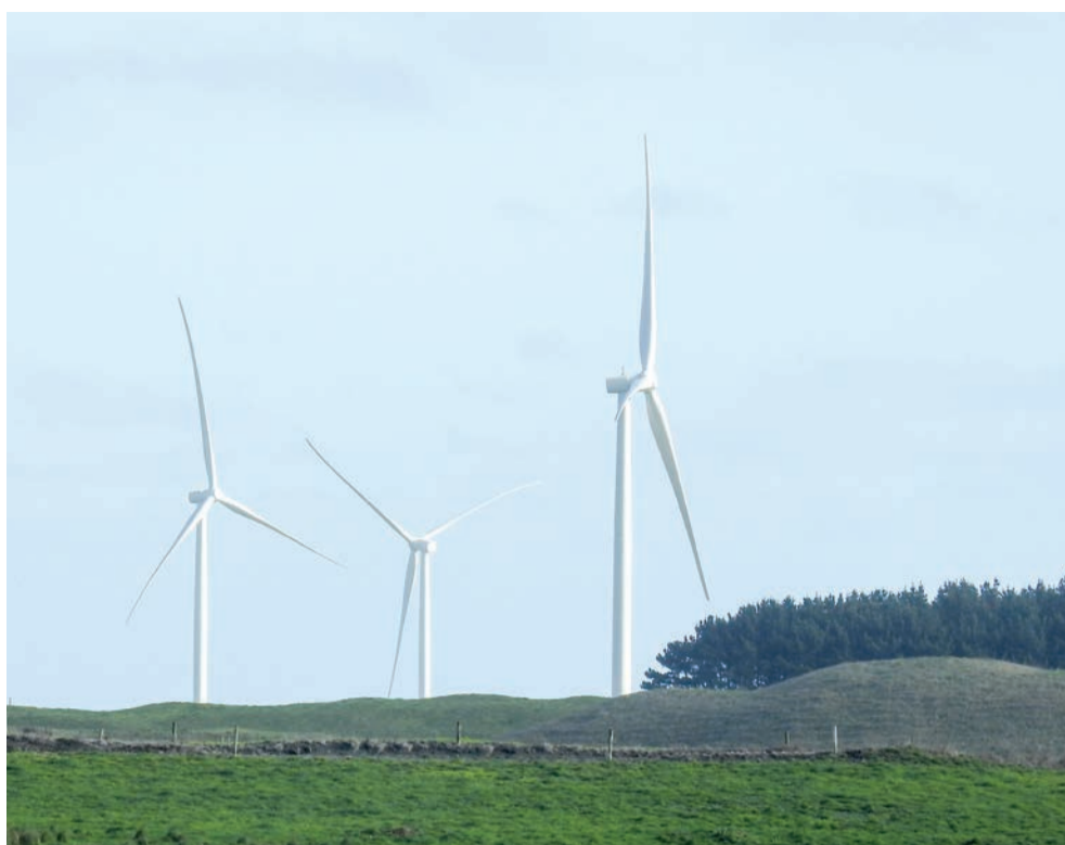
Work is progressing on a windfarm containing the country’s largest wind turbines.
